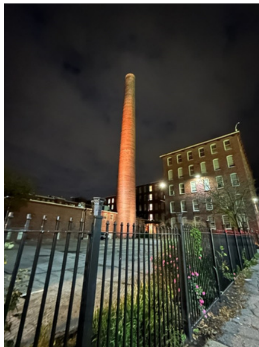
Test lighting of the Wannalancit Mill smokestack.
