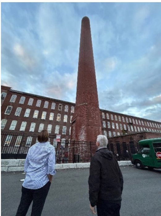
The LWVI team tours at Mill No. 5 during a recent tour of buildings and smokestacks downtown.
